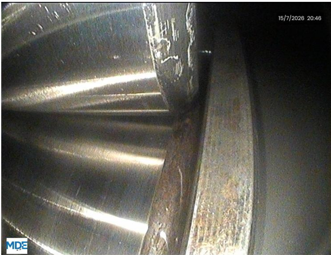
Photo 6: Output shaft, non-driven end. No deviations have been observed.
