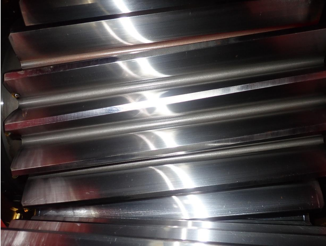
Photo 1: Input shaft, pinion. No deviations have been observed.
