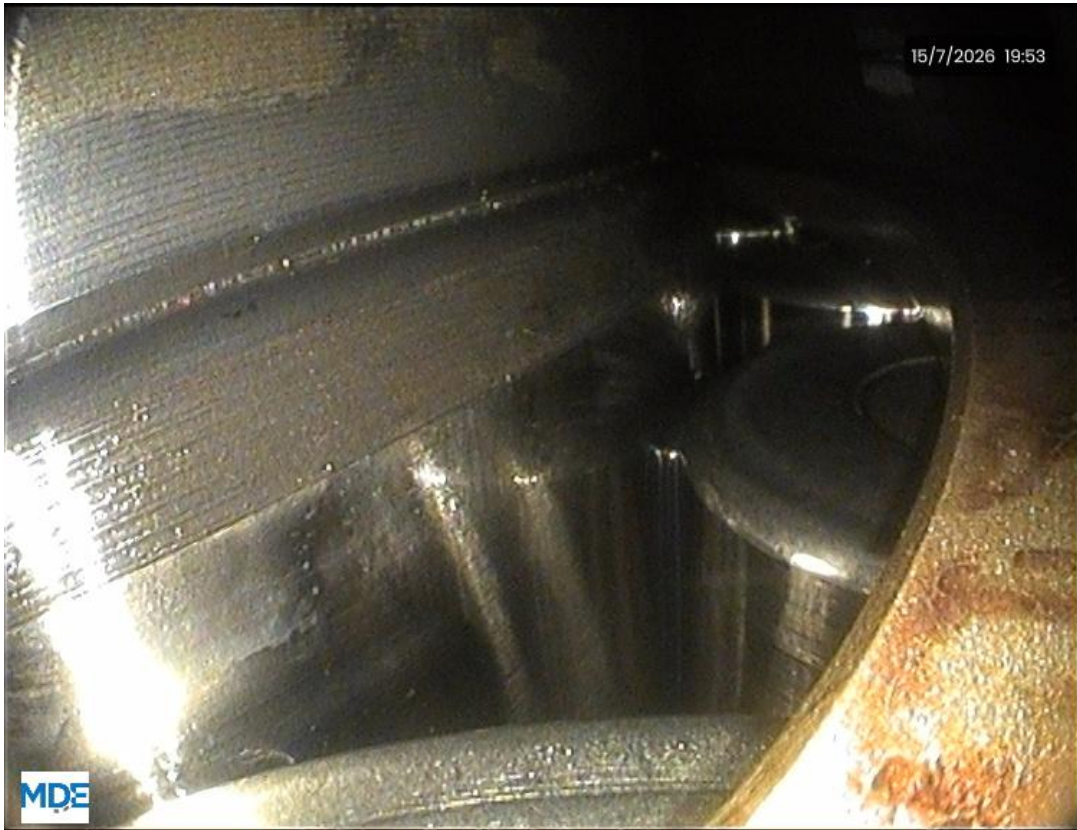
Photo 11: PTO non-driven end. No deviations have been observed.
