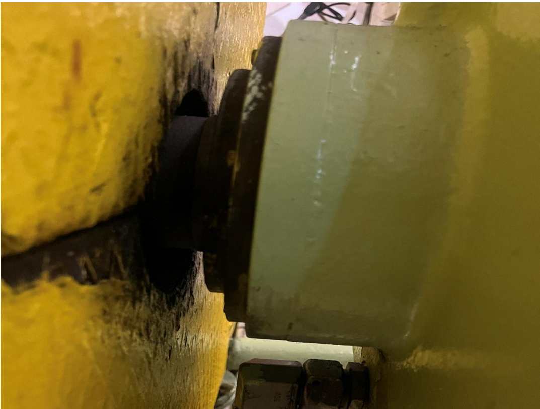
Photo 4: PTO shaft. No leakages have been observed.
