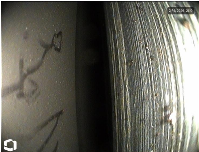
Photo 29: Coil 50. Debris and paint damage
