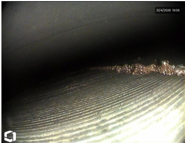
Photo 1: Coil 22. Debris and paint damage.
