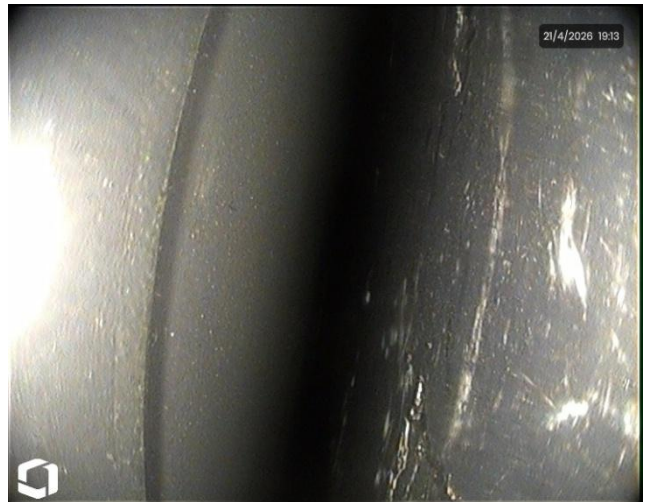
Photo 2: Coil 23. Debris and burn surface.
